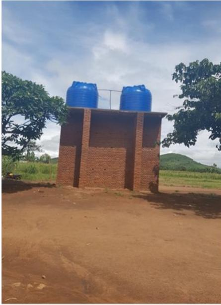
St. Lawrence water project included the drilling of the borehole, installing an electric water pump, building a pump house, installing a solar energy system connected with the electric pump, building a supporting frame holding two 5000-liter water tanks and installing an underground pipeline system. The work was implemented by Niho Systems from 4 November 2019 to 10 February 2020. The total amount of the project was **EUR 12,839.44**, which was equivalent to 10,464,143.60 Malawian Kwacha.
